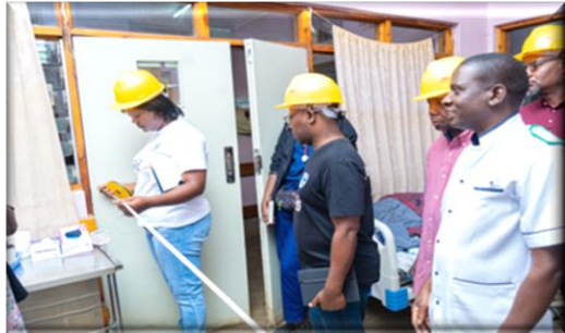
MK90 Million towards expansion and renovation of Zomba Central Hospital Maternity Ward High Dependency Unit.
